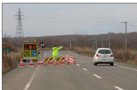
(a) Roadway worksite
