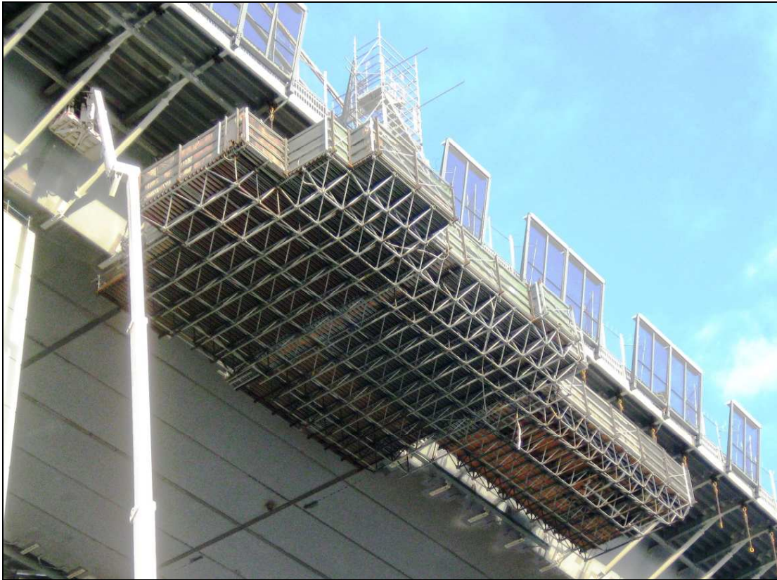
Closer view of one of the suspended work platforms
