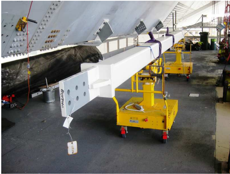
Cantilever bridge section prop transporters
