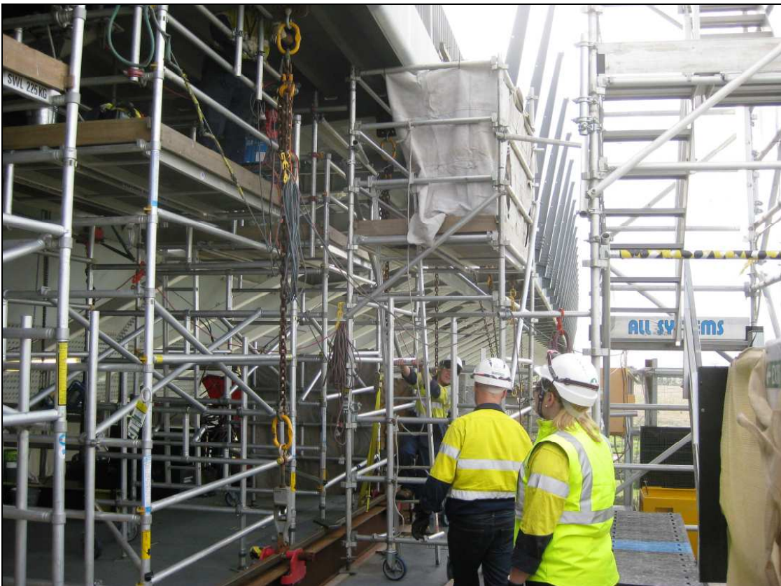
View inside one of the suspended work platforms
