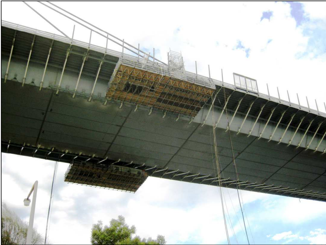
View of suspended work platforms
