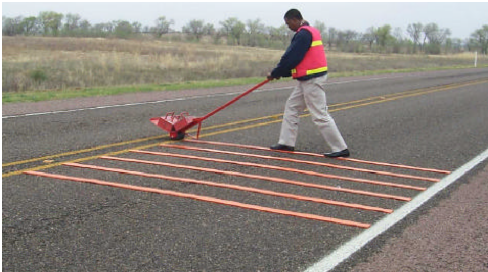
FIGURE 2 Rumble strip installation
