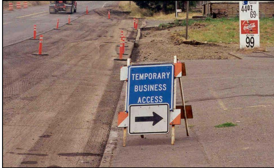
FIGURE 2 Business Access sign with directional arrow mounted on Type II barricade.
