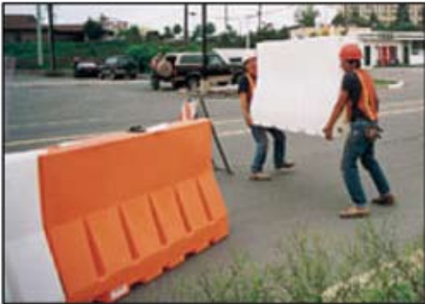
Figure 3. Empty Ballast-Filled Barrier Segments
